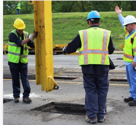
Flood Protection Drill - Assembling Stop Log Structure
