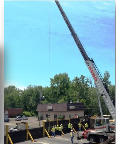
Flood Protection Drill - Assembling Stop Log Structure
