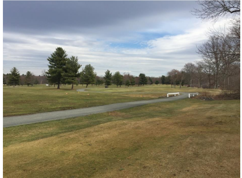
Refurbished Cart Paths
