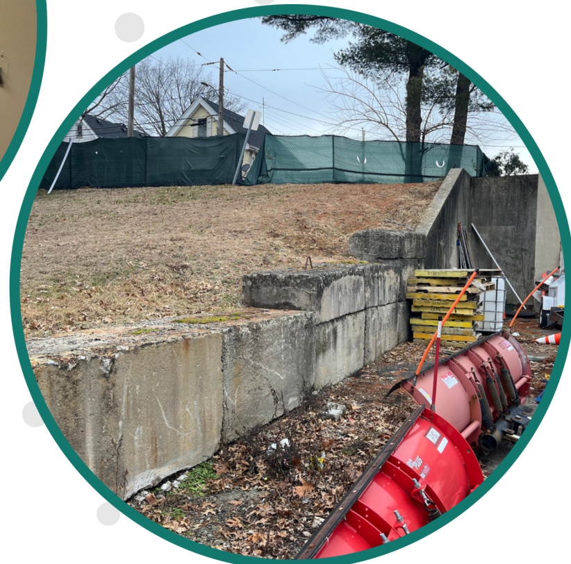
current retaining wall
