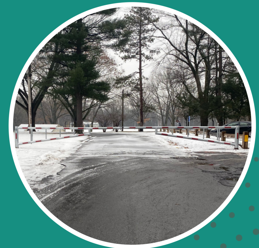
Martin Park gate and guard rail
