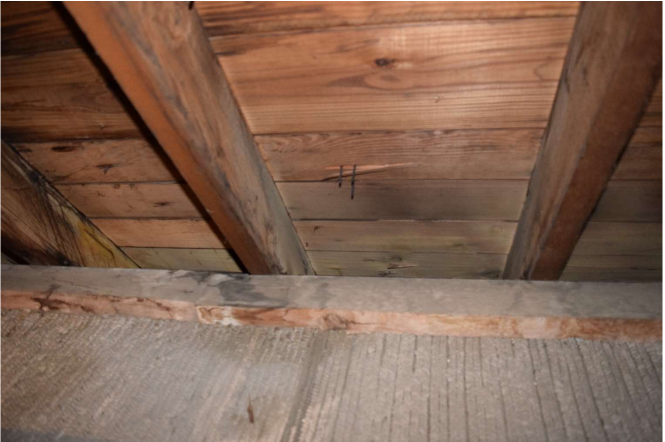
Photo A11 – North Wing Attic Looking towards west.
