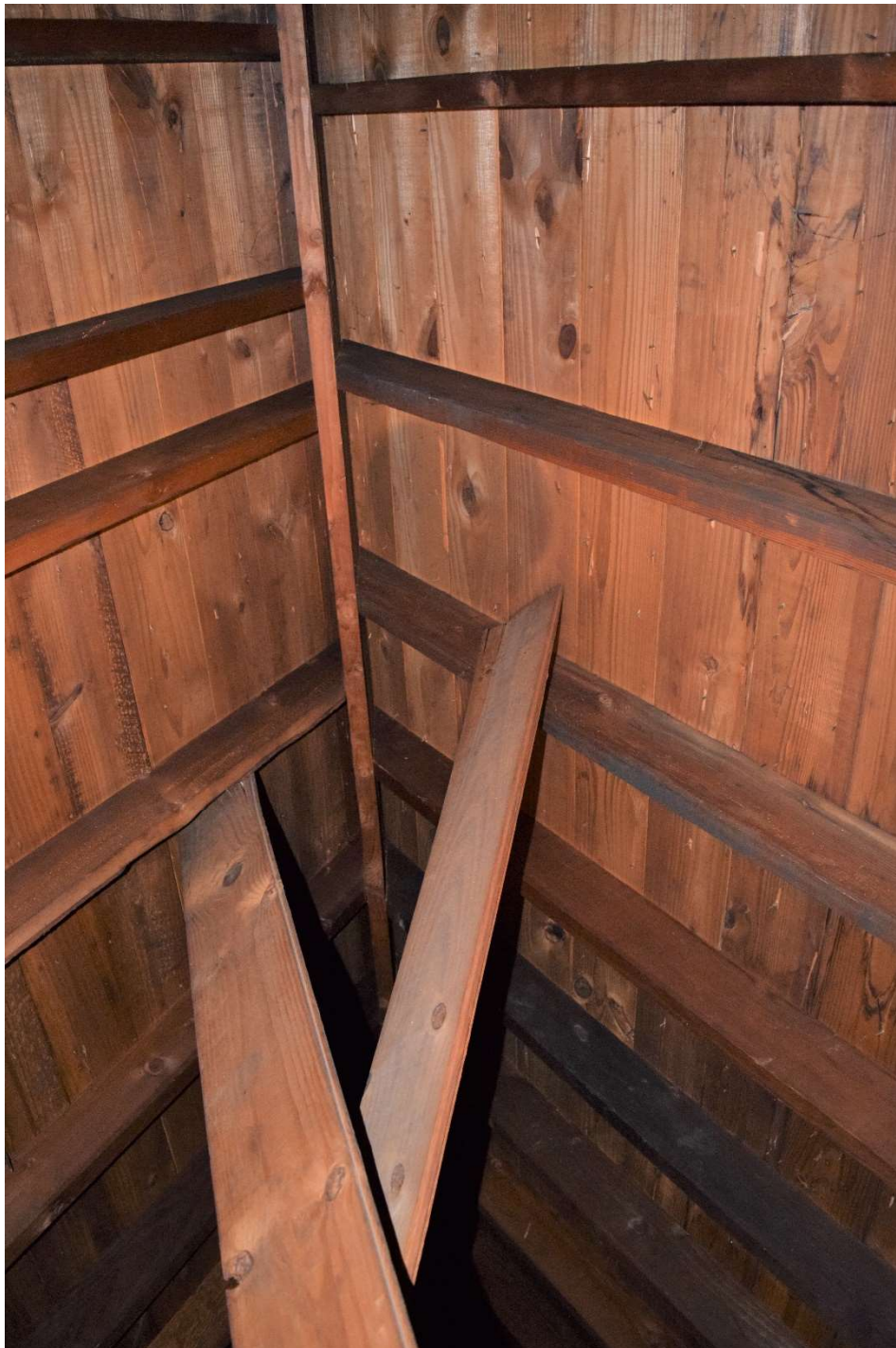
Photo A6 – North Wing Attic
