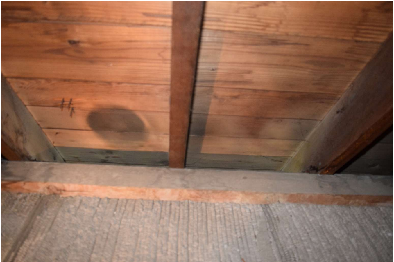
Photo A10 – North Wing Attic Looking towards west.
