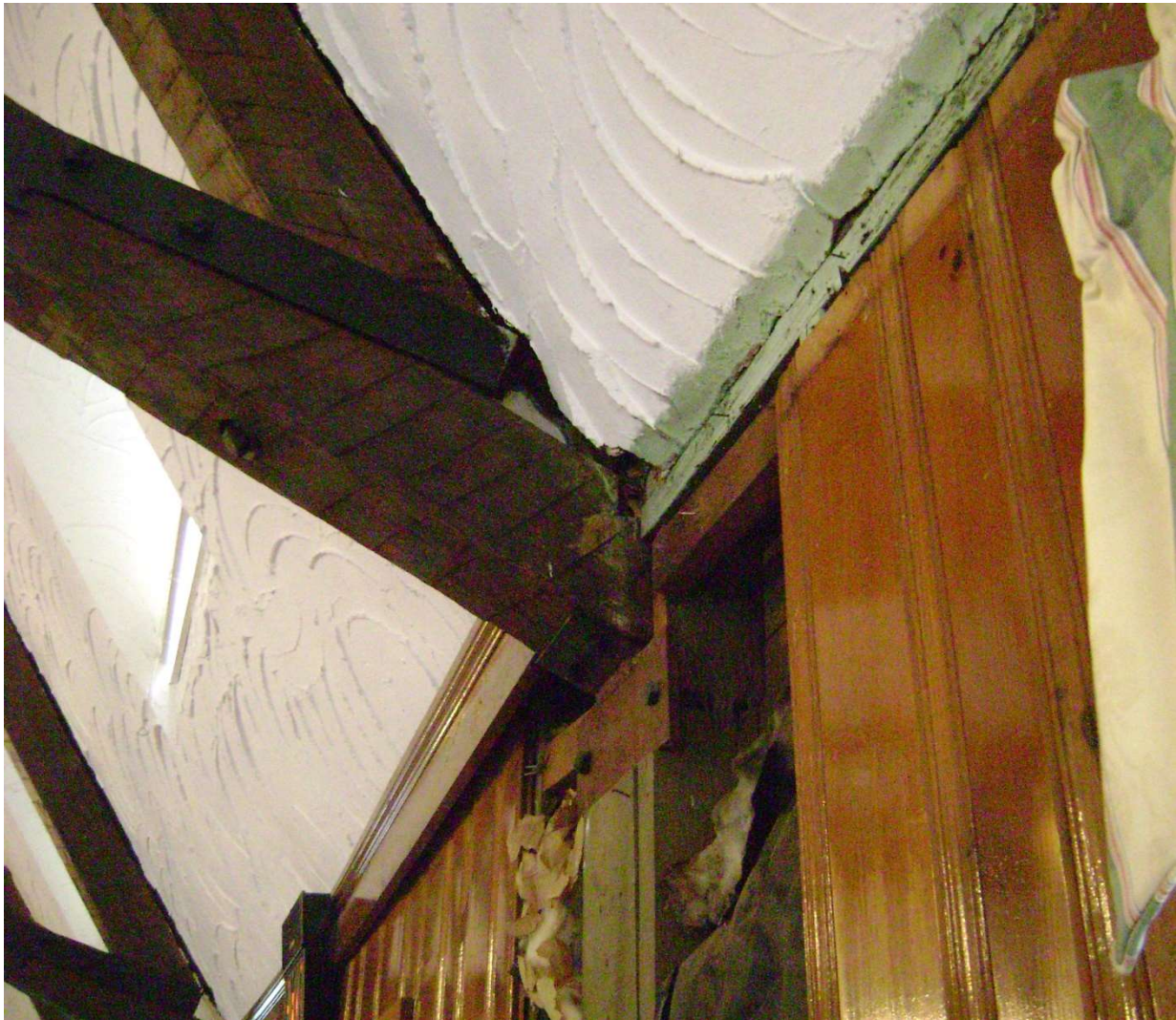
Photo EW3 – North Wing Ballroom Truss connection to wood column.
