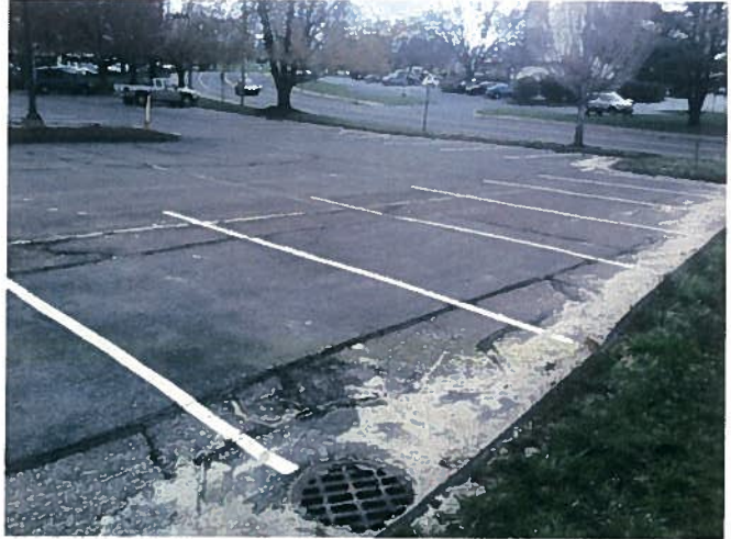
MH9b location. Parking lot looking northeast
