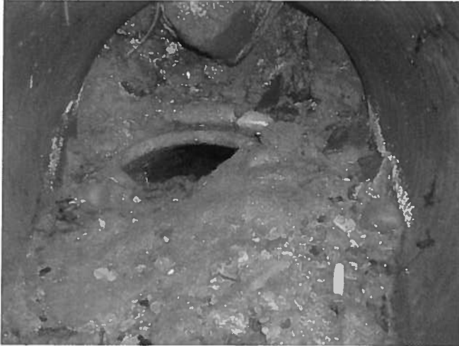
MH9b – 8-inch-diameter VCP to MH9.
