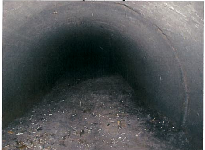
MH9b looking towards MH8.
