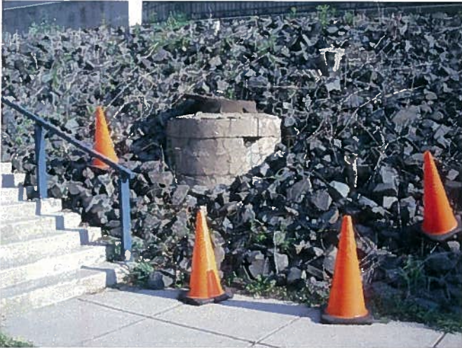
Founders Bridge Manhole location
