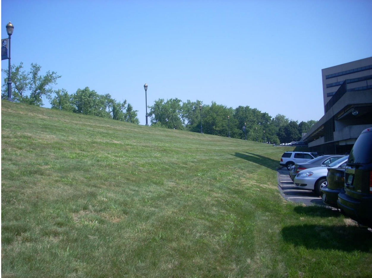
Photo looking North (north of Founder Bridge) to northern terminus of project. Toe drain replacement proposed for levee toe area to left of paved parking area.
