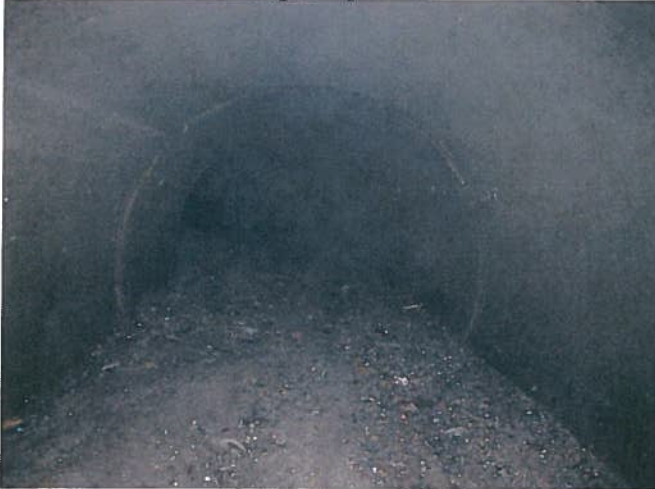
MH9b looking towards buried manhole.
