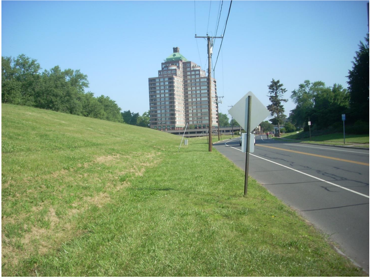
Photo looking North. Toe drain replacement proposed for levee toe area to the left of paved street (East River Drive)
