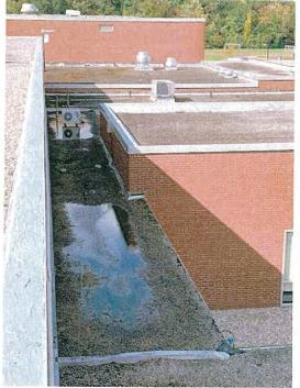
storm. Perimeter flashings have been coated several times over the years in an attempt to exend their life and stop leaks. While it is a very large expense to re-roof the entire school, doing so will ensure the intregrity of the building and safety of the occupants for years to come.
