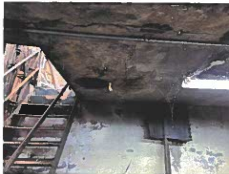
Failing Concrete Floor Slab and Concrete Encased Steel Beam
