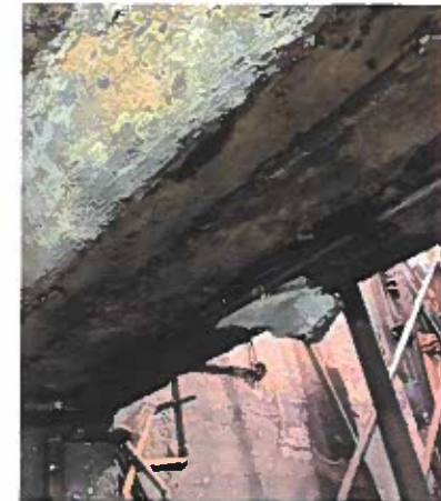
Failing Concrete Floor Slab and Concrete Encased Steel Beam
