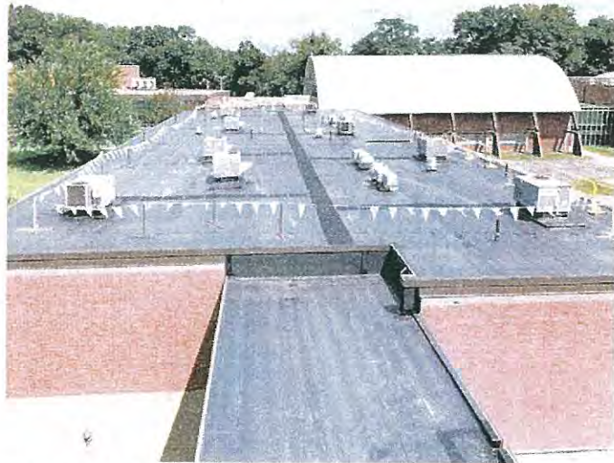
Example of new EPDM roofing system "C" Building – completed in 2019
