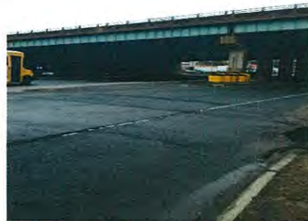
Figure 15. No Crosswalk on Ramp
