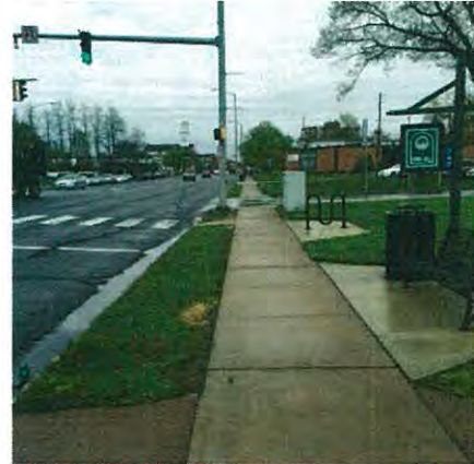
Figure 8. No Pedestrian Signal at the Intersection of Town Hall and Main Street
