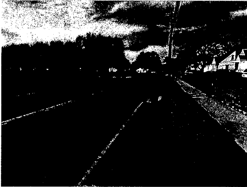
106 GOODWIN STREET FACING WEST
