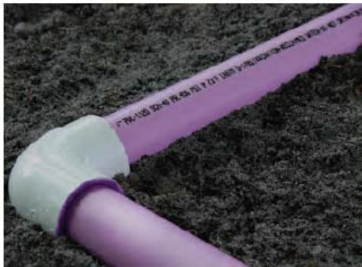
Purple piping is required for nonpotable water distribution.
