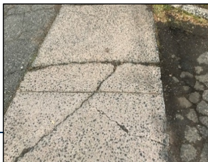
Cracked Sidewalk on Silver Lane
