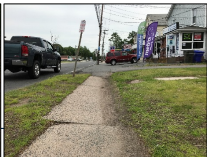
Uneven and Sloped Sidewalk
